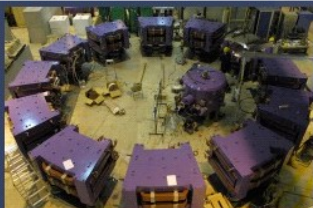
150-MeV Proton FFAG Under construction at KEK
