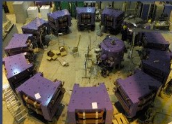
150-MeV Proton FFAG Under construction at KEK
